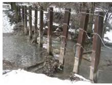
Photo 4: Debris structure west of main bridge.
