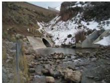
Photo 15: Outlet of Parley's Creek culvert (left side), highway drainage culvert (above it) and outlet of Terminal Reservoir (right side).
