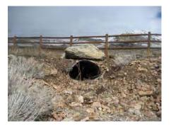
Photo 14: Outlet of third 48" Culvert.
