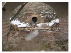
Photo 12: Two culverts for routing offsite runoff through the park. The top of the second, buried corrugated metal pipe is visible inside the archway.
