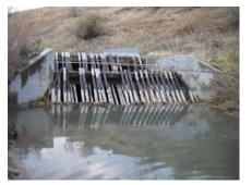
Photo 5: Debris structure at west culvert inlet.
