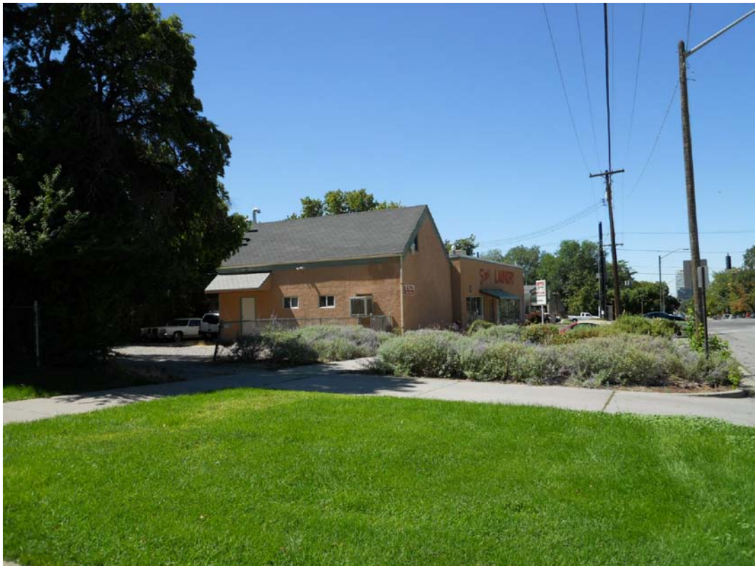
300 South (looking west from driveway)
