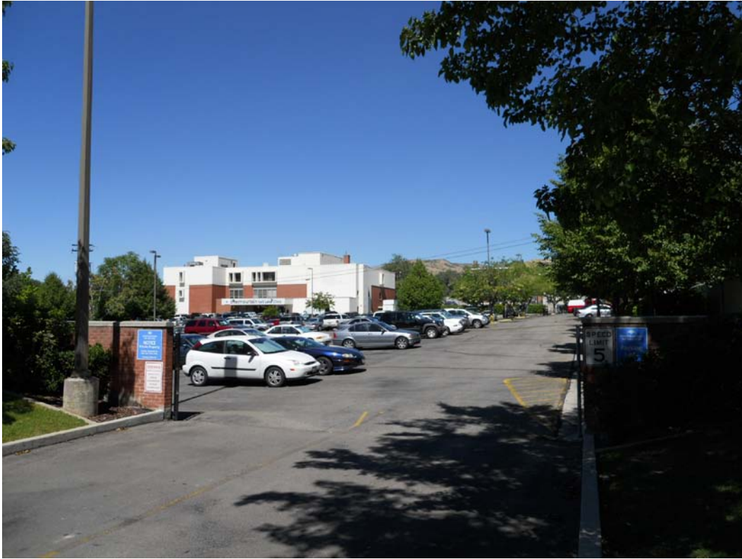
400 South (site of western drive – looking at existing clinic)
