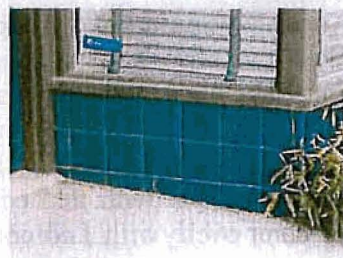
An example of an original tile bulkhead at 422-426 North 300 West Street.
