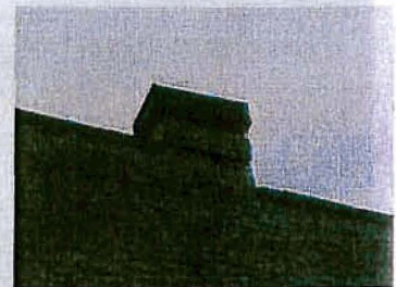
Original chimney, 68 North K Street.
