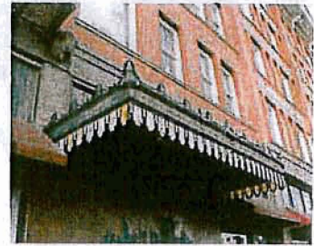
An example of a metal awning at 379 South Main Street.
