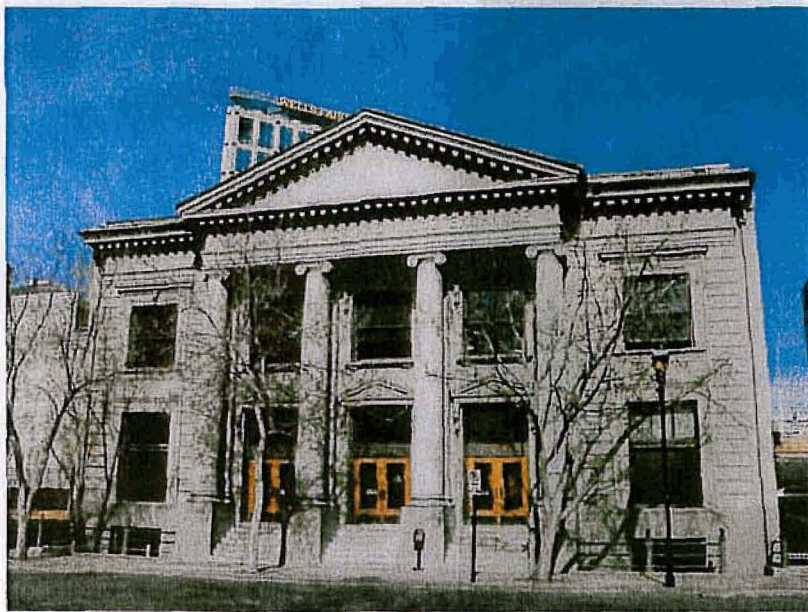
The Salt Lake Stock and Mining Exchange at 39 Exchange Place was built in 1908 and it retains much of its original design. The building's form is central block with wings while its architectural style is Neo-classical. The projecting central bay displays Ionic columns and a large pediment with modillion blocks.
