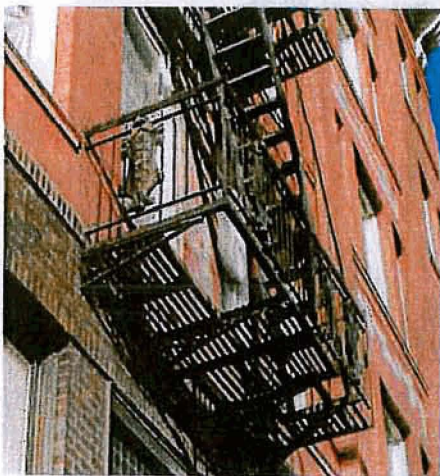
Proper fire escape placement at 379 South Main Street.
