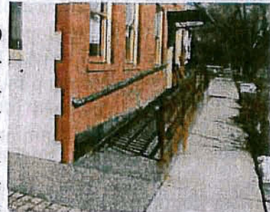
An appropriate access ramp at 569 2nd Avenue North.
