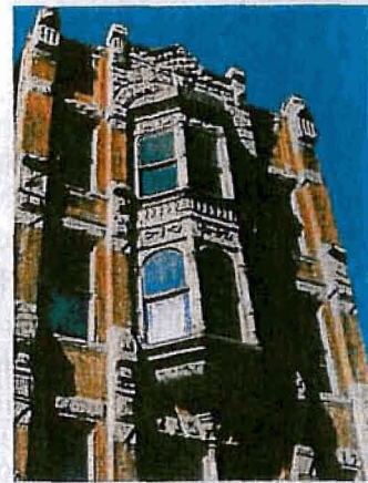
Historic masonry adds distinct character to buildings and should be preserved and maintained with proper care. (328 South Main Street)
