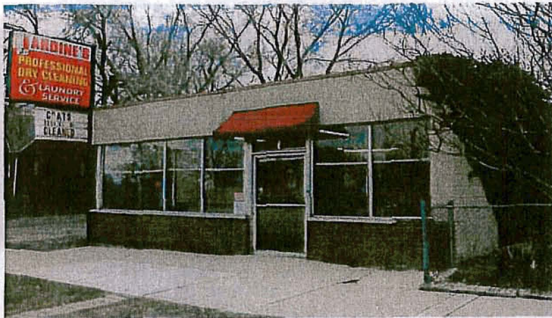
Many neighborhood commercial buildings were built with poured concrete pavement extending the width of the storefront. This example is at 442 North 300 West.
