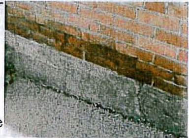
A concrete foundation at 422-426 North 300 West Street.
