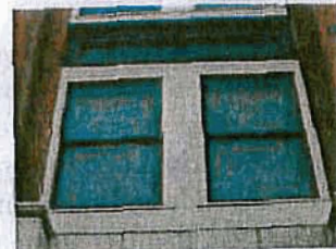
These one-over-one sash windows at 372 200 South are a good example of replacement windows. They match the historical design and configuration of the original windows.
