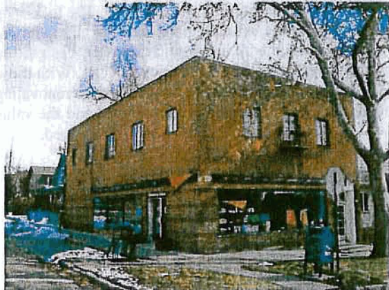
This building was designed with simple detailing ca. 1930 and has rectangular steel casement windows and original display windows (702 E. K Street).
