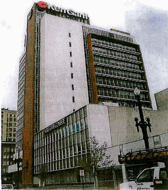
The First Security Bank Building at 405 South Main Street was built in 1955 and features an exterior curtain wall of glass, aluminum, and enameled porcelain panels.
