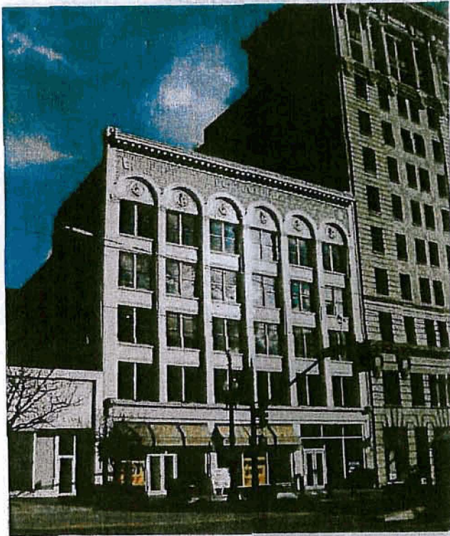
The Felt Building at 335-339 South Main Street was constructed in 1909 and has a separate storefront zone and unified upper façade. The building is distinguished by its glazed terra cotta and arched panels below the cornice.
