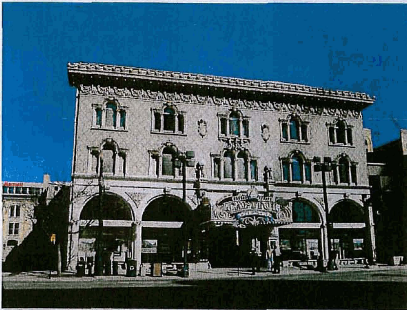
The Orpheum (Capitol) Theatre at 42 West Second South Street was built in 1913 and reflects the arcaded block building type and Renaissance Revival architectural style. The building displays polychrome terra cotta on the main façade and has been restored into a multi-use theater building.
