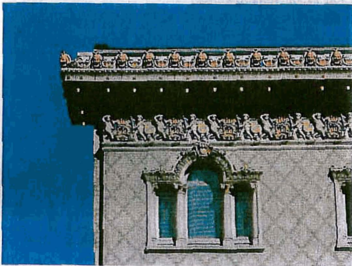
Architectural details of the Capitol Theater include an ornate cornice and decorative window hoods and surrounds.
