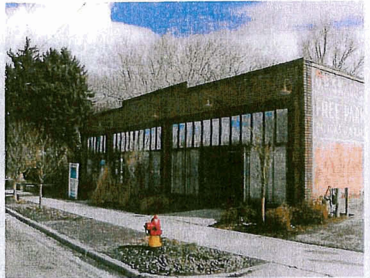
The building at 422-426 N. 300 West has been well preserved and retains much of its original storefront.
