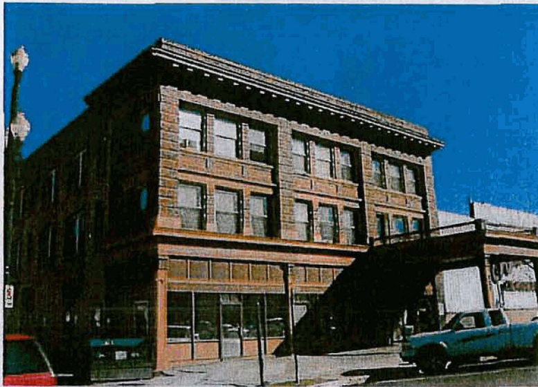
Pilasters divide the upper façade at 222 West Third South Street and present a balanced and symmetrical appearance.
