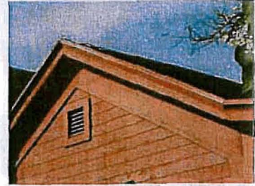
Maintain historic roof shapes (271 Center Street).
