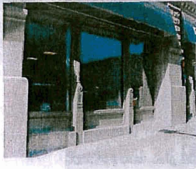
Cast Iron columns at 268 South State Street.
