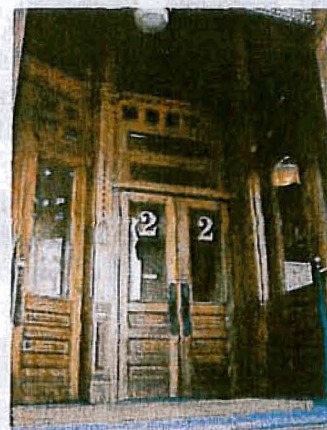
Original wood doors at 22 100 South.
